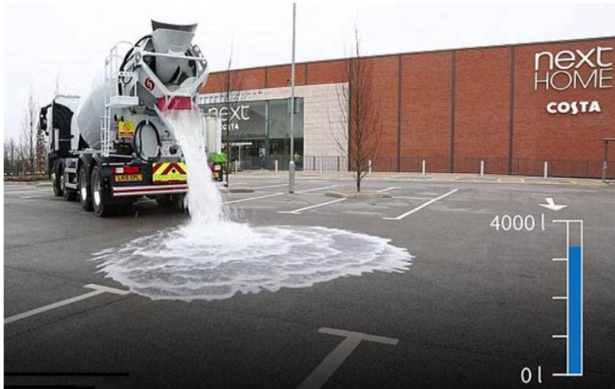
Topmix Permeable concrete is said to be ideal for car parks where standing water and puddles can be a problem. Photo: Lafarge Tarmac.
